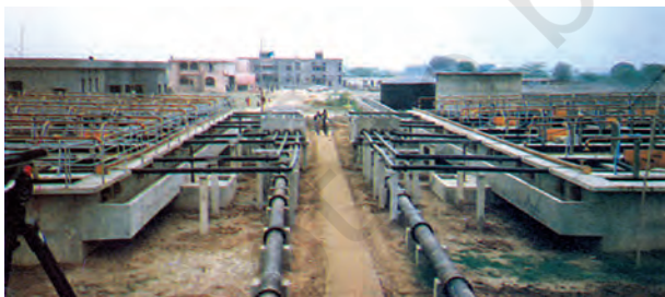
Fig. 6.10: Sewage Treatment plant under Yamuna action plan at Faridabad
