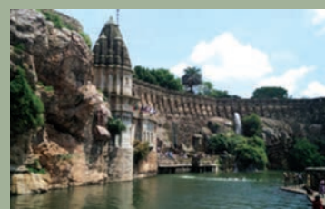
Fig. 4b. Chittorgarh Fort, Rajasthan
